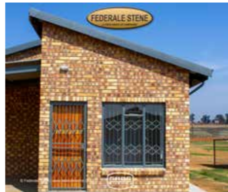
SEMIFACE TRAVETINE PROJECT: HOUSING DEVELOPMENT | SEMIFACE (FBA)
