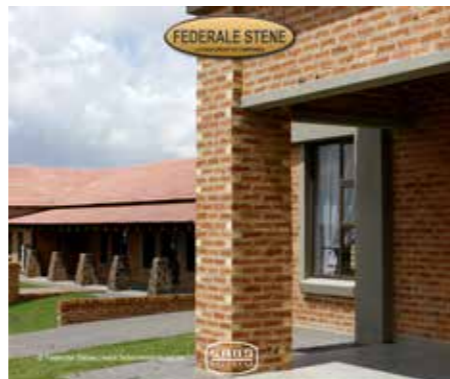
ROOIBOS TRAVETINE PROJECT: TERRA NOVA RETIREMENT VILLAGE | FACEBRICK (FBS)
